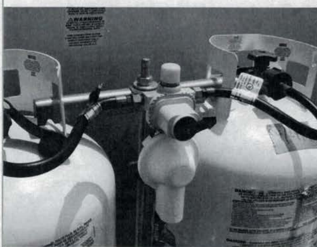
Figure 5-49 Automatic Changeover Regulator Indicator
