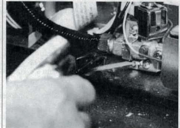
Using solution to check for leaks
